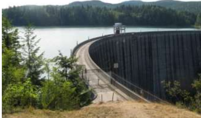
Alder Dam by Basia Irland
