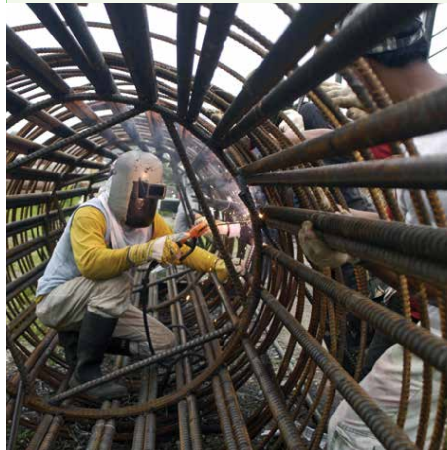
Construction in Philippines. Image: Nonie Reyes, World Bank.
