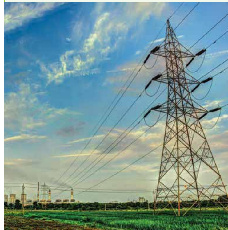
Wanakbori thermal power station, India. Image: Dhruv Patel.
